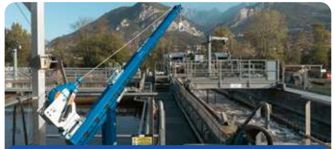
Confined space tank
